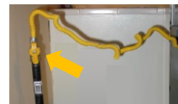
Location of valves for meter (above) and appliance supply line (below)
