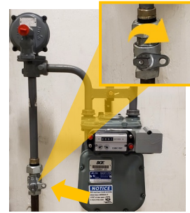
Location of valves for meter (above) and appliance supply line (below)
