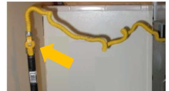
Location of valves for meter (above) and appliance supply line (below)
